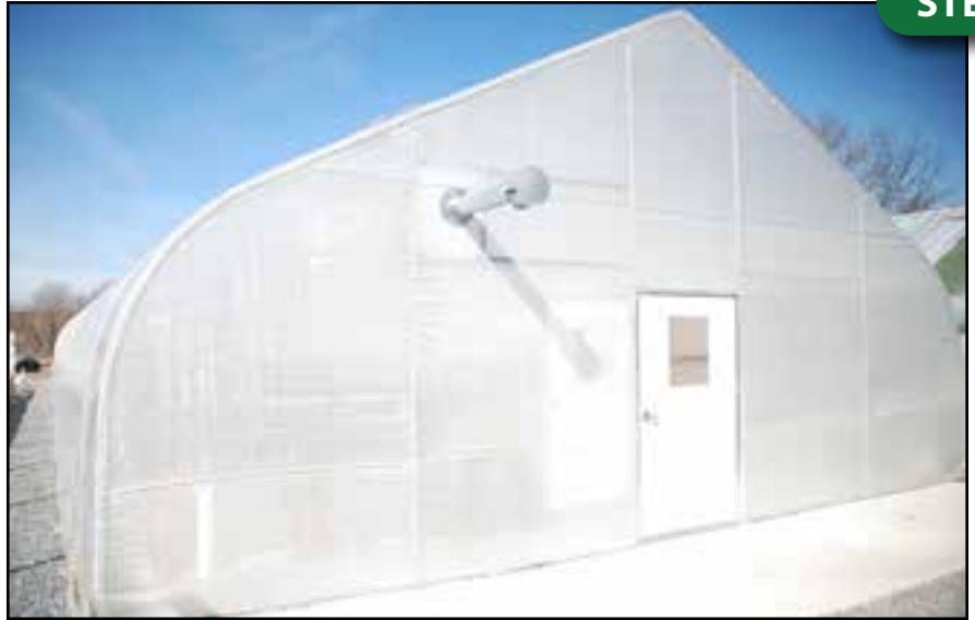
Greenway Farms | Hackettstown, NJ The end wall shown has a “No-Thrip” insect screen.
