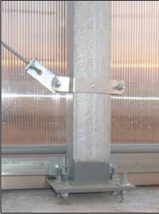
This photo shows a column with a base plate mounted on a concrete wall.
