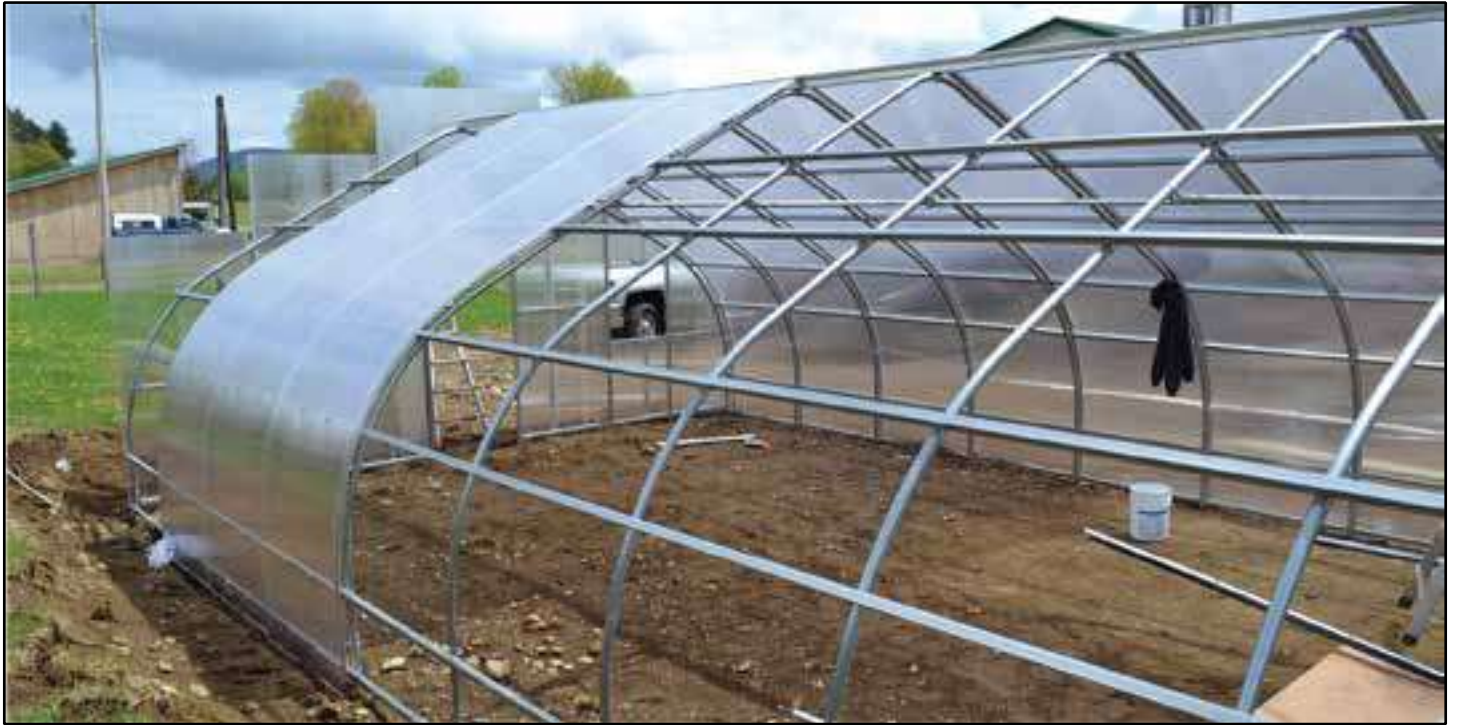
Polycarbonate installation on a roof.
