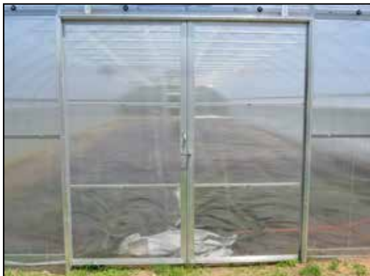
Double sliding doors with polycarbonate panels.
