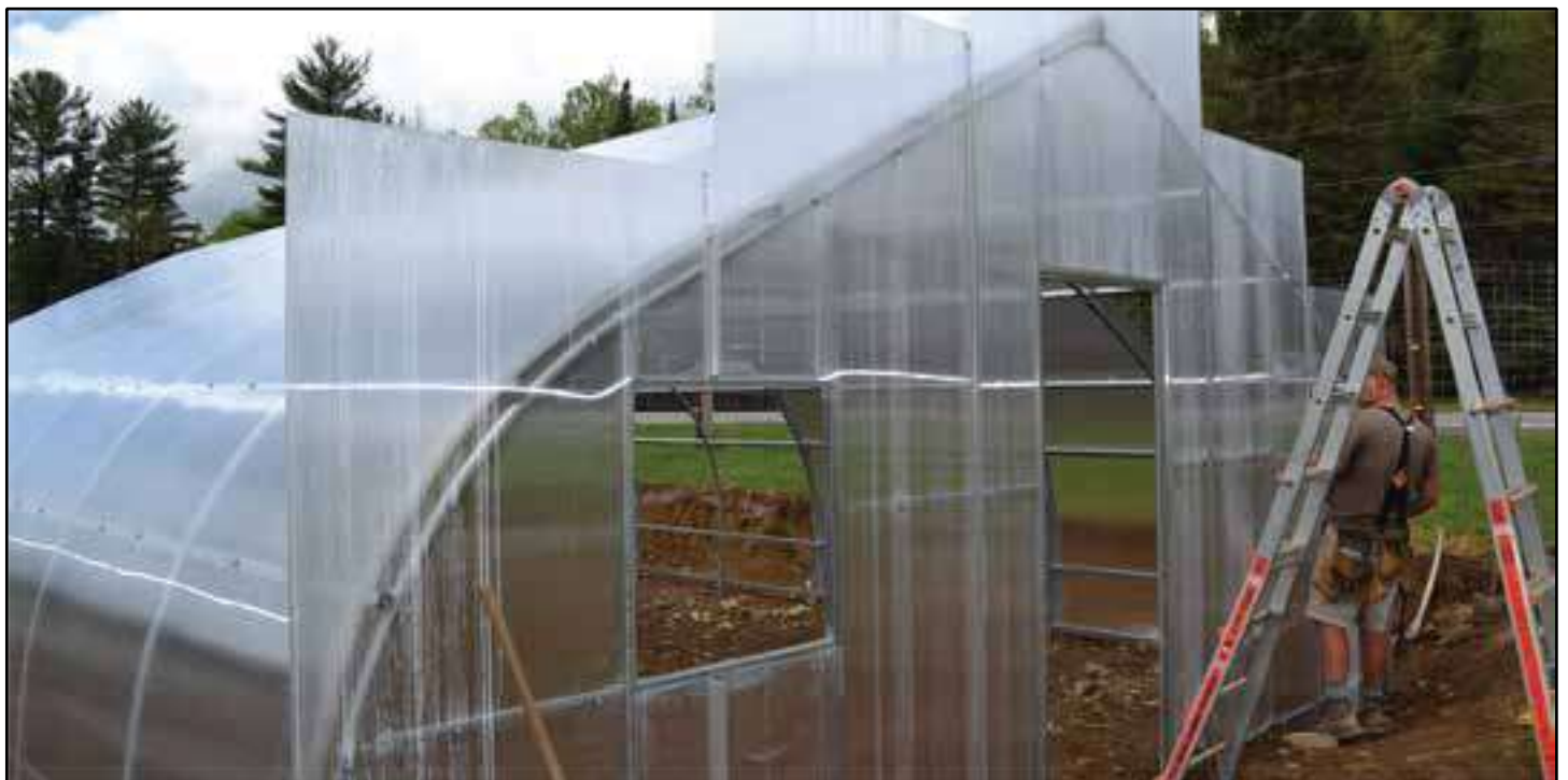
Polycarbonate installation on an end wall.
