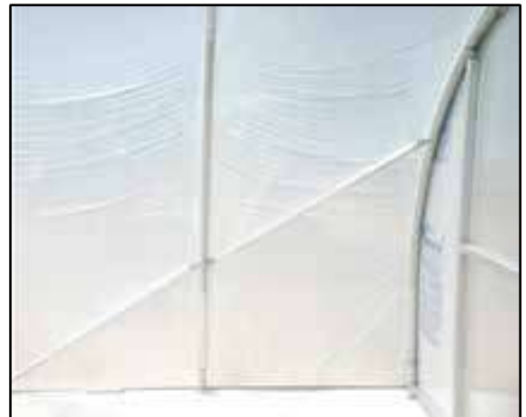
Wind bracing shown.
