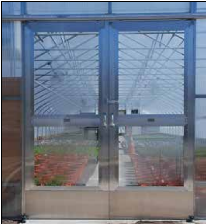
Double sliding doors with clear vision glass panels.
