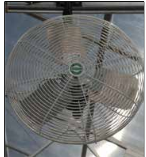
20" fan recommended for larger greenhouses and for maximum air circulation.
