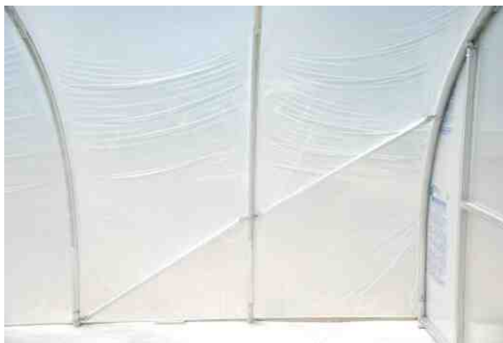
Standard wind kit bracing shown.
