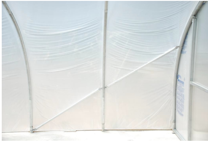
Standard wind kit bracing shown.
