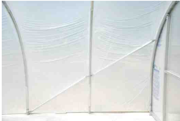
Standard wind kit bracing shown.
